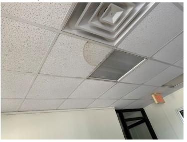
Ceiling- Acoustical Tiles show water damage.
