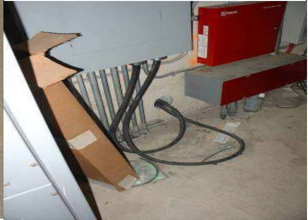
8. Typical Distress: NEC Art 400 Violation – Portable Cord Used as Permanent
