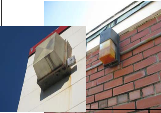
1. Typical Distress: Stained Lens (Exterior)
