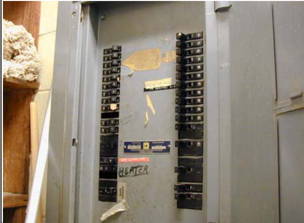
9. Typical Distress: Missing Panel Cover
