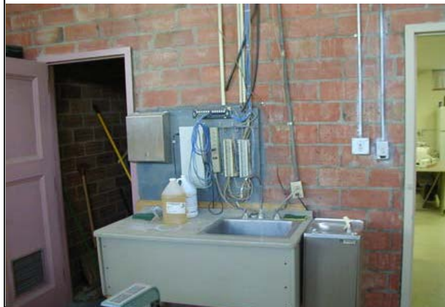
11. Typical Distress: Code Violation – Panel & Non-GFCI Outlet at Sink and for Water Cooler
