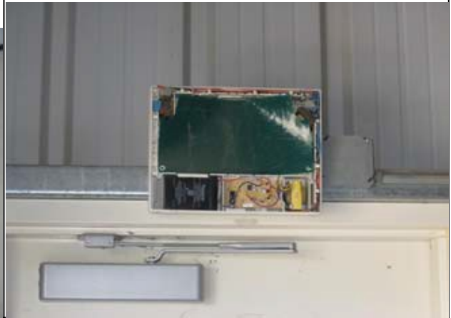
4. Typical Distress: Missing Exit Sign Face
