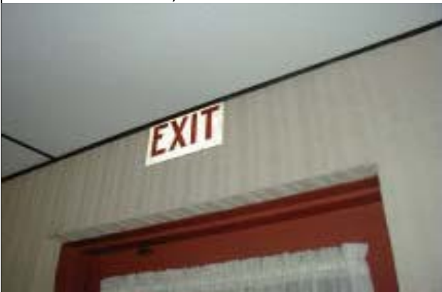
3. Typical Distress: Non-Compliant Sign, Locally Made, No Power Source
