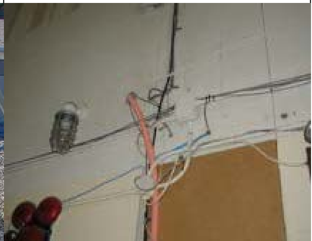
10. Typical Distress: Surface Mounted Electrical Wiring not in Conduit
