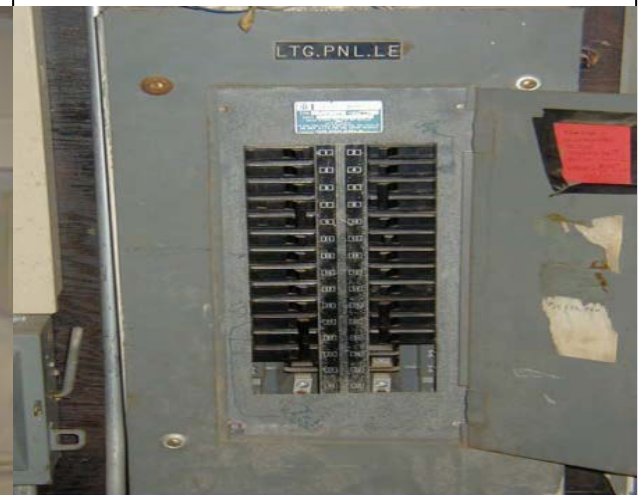
6. Typical Distress: Exposed Bus Bars
