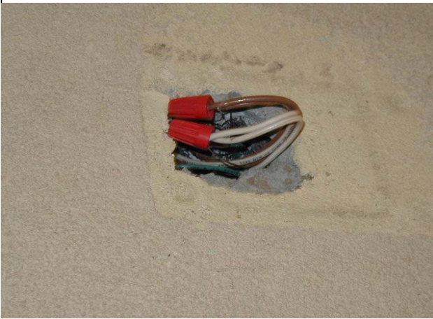
7. Typical Distress: Exposed Wiring on Exterior Wall
