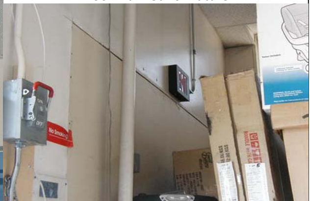
6. Typical Distress: Exit Sign with no Door – Door Planned for Future
