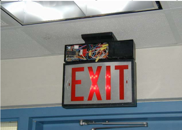
5. Typical Distress: Exit Sign with Exposed Wiring
