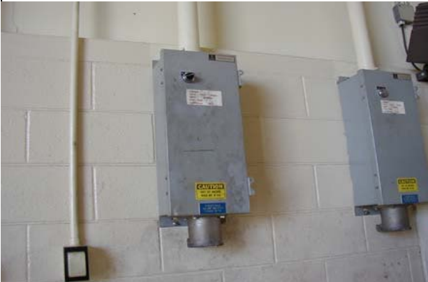
7. Typical Distress: Arc Faulting 440V Receptacle
