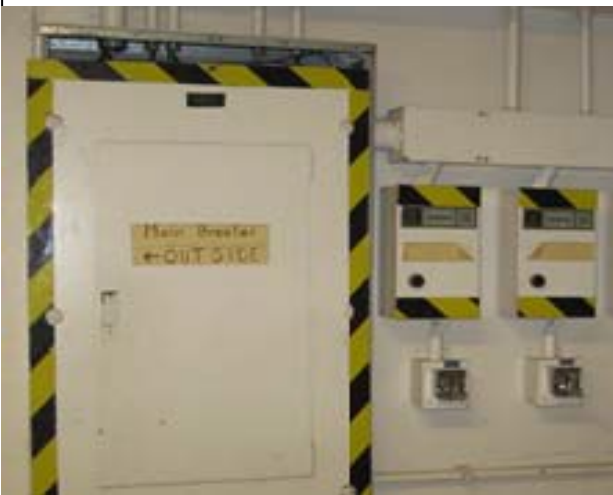
5. Typical Distress: Modified Panel, Exposed Wiring
