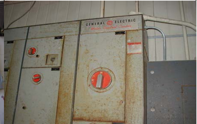
8. Typical Distress: Corroded MDP
