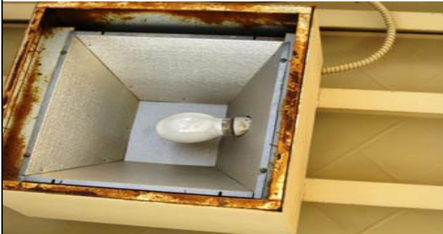
11. Typical Distress: Missing Lens, Corroded
