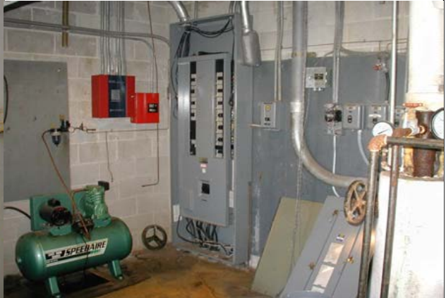
10. Typical Distress: NFPA 70 - Inadequate Working Space Clearance
