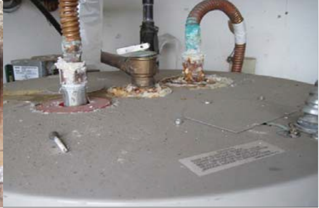
4. Typical Distress: Corroded
