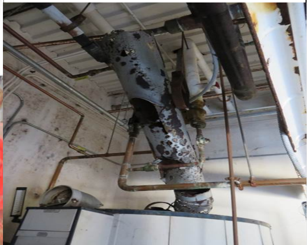
2. Typical Distress: Failed Water Heater Flue Vent Gas Vapor Accumulation in Mechanical Room
