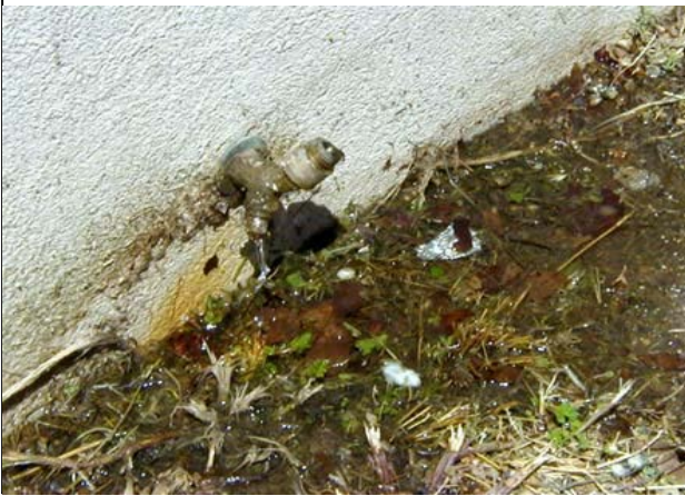
6. Typical Distress: Water Heater PRV not Correctly Plumbed
