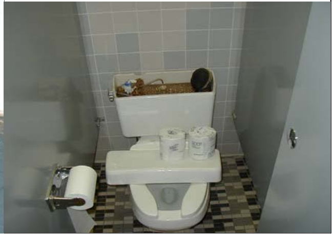
6. Typical Distress: Operationally Impaired – Broken Valve
