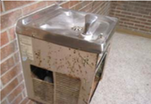
3. Typical Distress: Corrosion, Missing Housing
