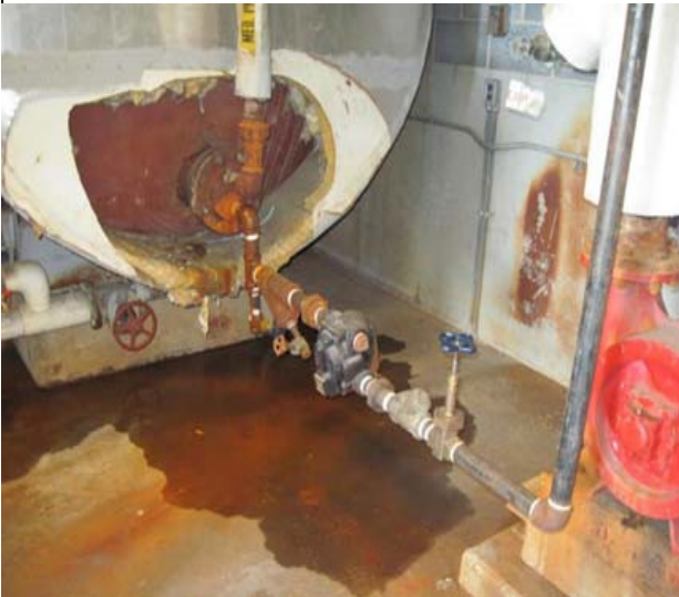
1. Typical Distress: Leaks, Insulation Missing
