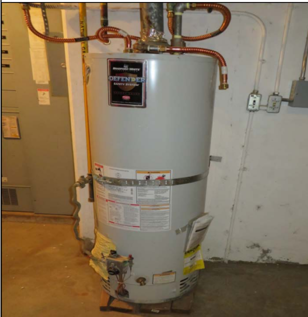
6. Typical Distress: Water Heater PRV not Correctly Plumbed
