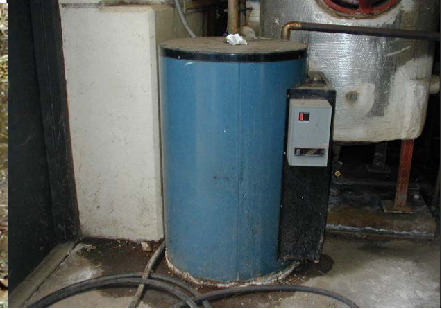
7. Typical Distress: Corroded & Leaking
