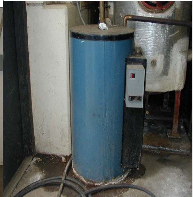
7. Typical Distress: Corroded & Leaking
