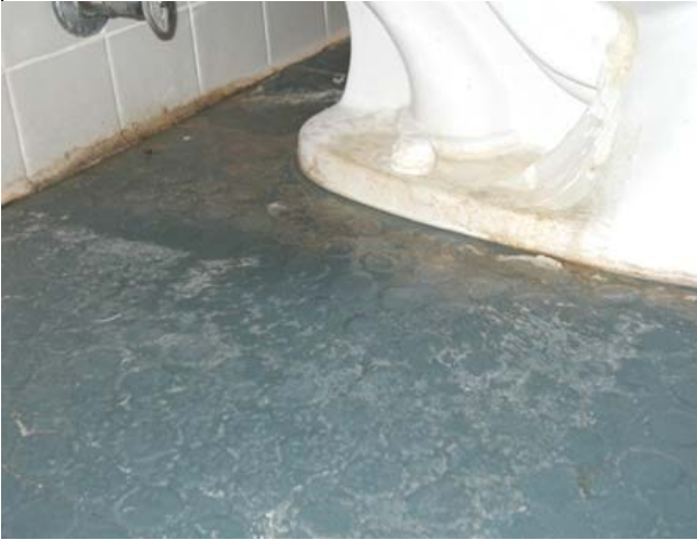
5. Typical Distress: Leaking Watercloset
