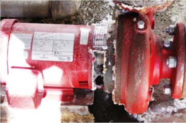
3. Typical Distress: Leaking Pump
