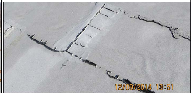
28. Typical Distress: Munition Storage Facility Earthen Covering Erosion
