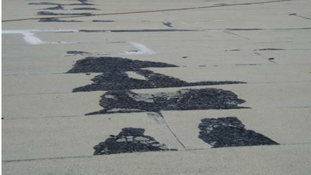
17. Typical Distress: Bubbling Asphalt Roof
