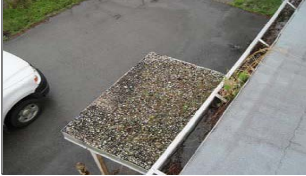
5. Typical Distress: Debris - Vegetation in Gutter
