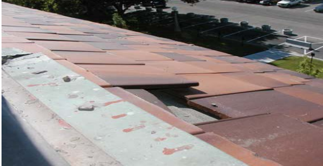
23. Typical Distress: Missing Roof Tiles
