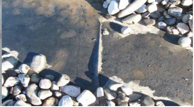
6. Typical Distress: Defective Seam
