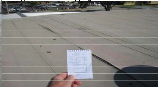
2. Typical Distress: Slipping
