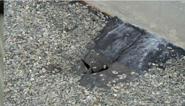
20. Typical Distress: Hole over Mechanical Room
