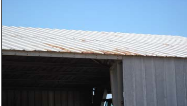
9. Typical Distress: Surface Deterioration
