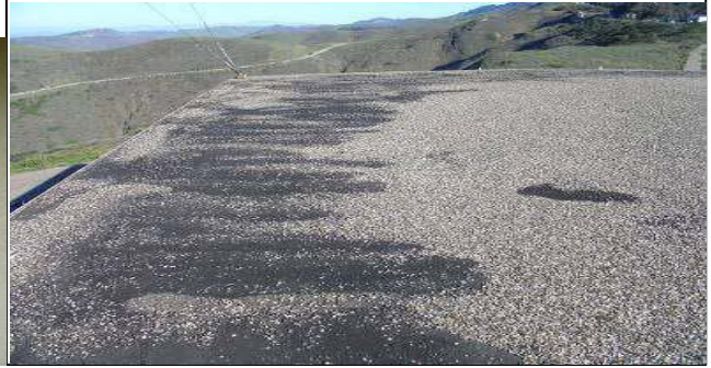
22. Typical Distress: Severe Wind Scour
