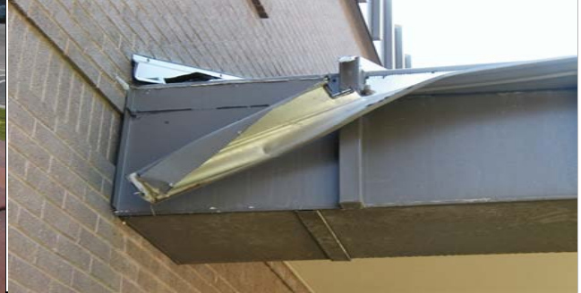
24. Typical Distress: Damaged Gutter
