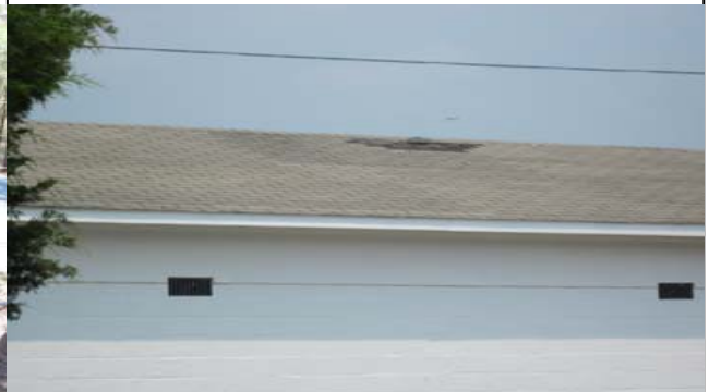
12. Typical Distress: Missing Shingles
