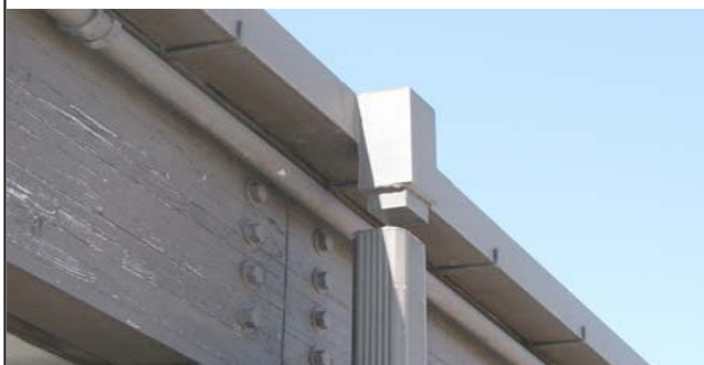
27. Typical Distress: Disconnected Downspout
