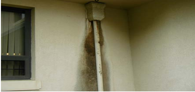
21. Typical Distress: Broken Downspout Staining Wall
