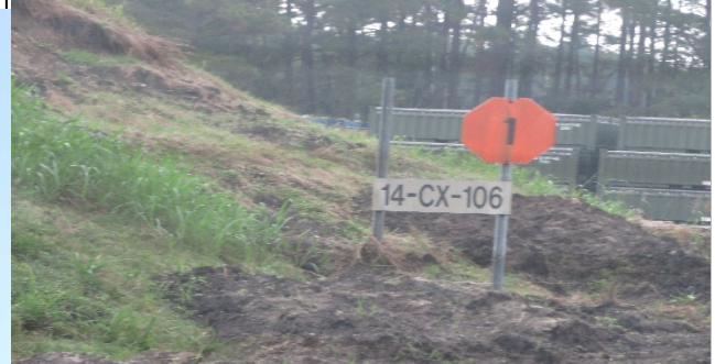
28. Typical Distress: Munition Storage Facility Earthen Covering Erosion
