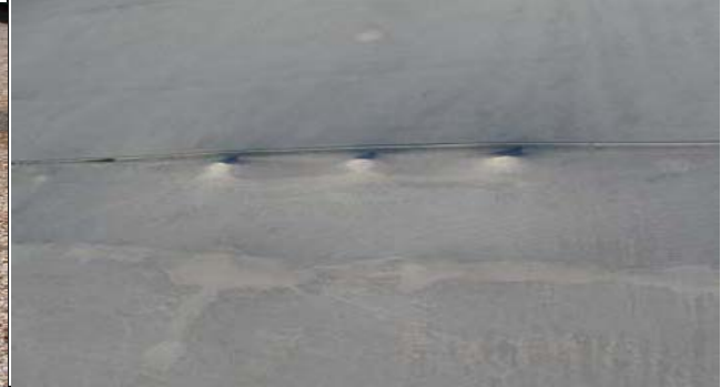
8. Typical Distress: Fastener "Pop-up"
