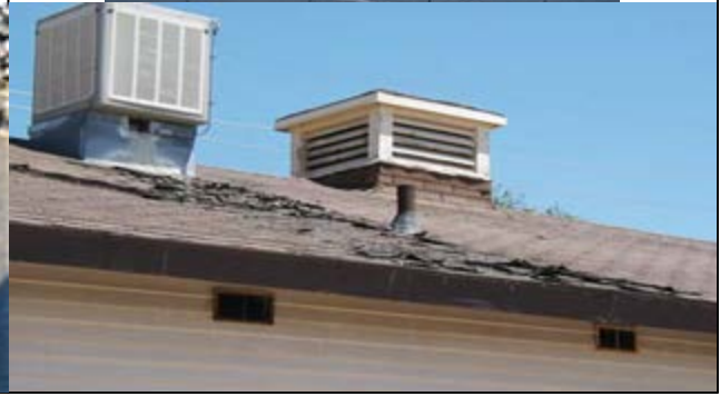
14. Typical Distress: Asphalt Shingles Curling
