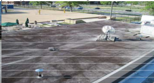
4. Typical Distress: Staining
