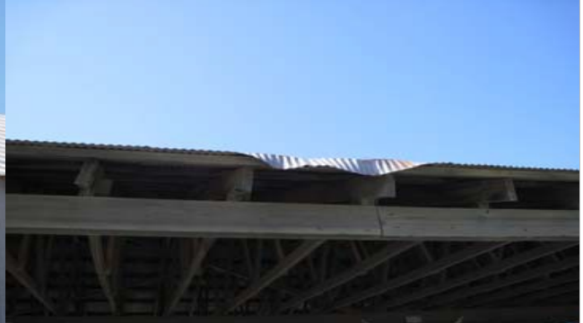
10. Typical Distress: Impact Damage
