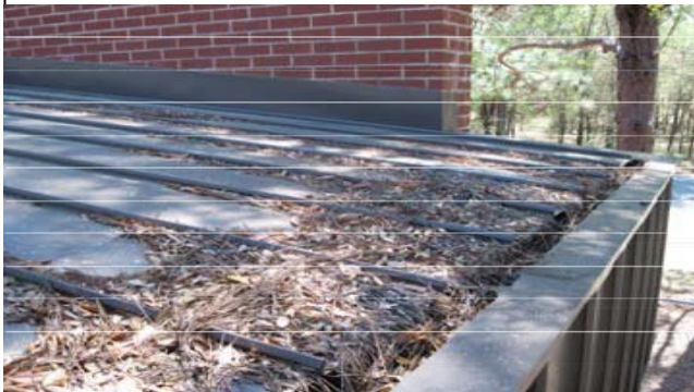
11. Typical Distress: Debris - Vegetation
