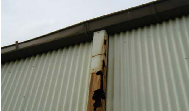
19. Typical Distress: Corroded Downspout
