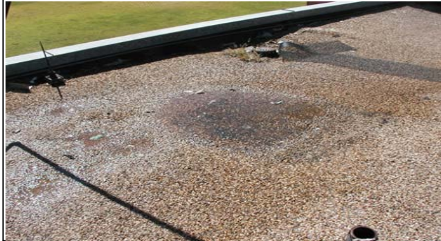
7. Typical Distress: Ponding
