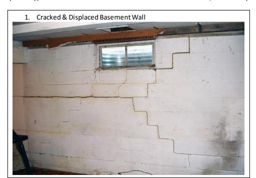
Examples of typical basement walls distresses or conditions include Cracks, leaks or displacement.
